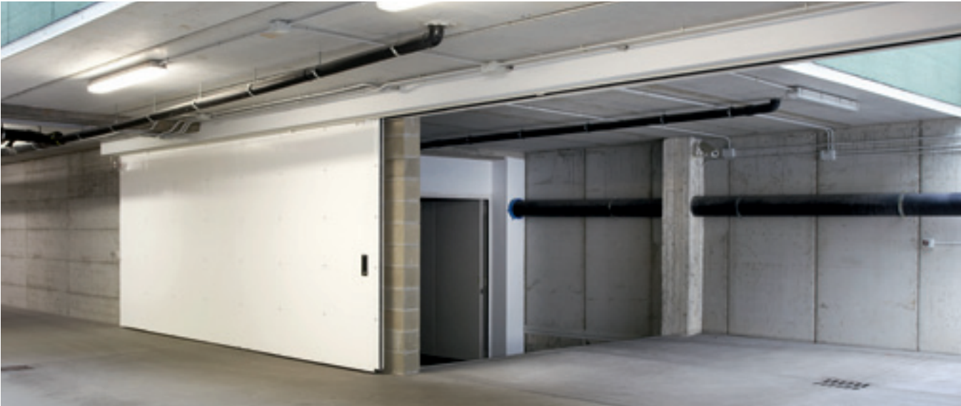
Portone tagliafuoco scorrevole Rolling Rolling fire rated sliding main door
